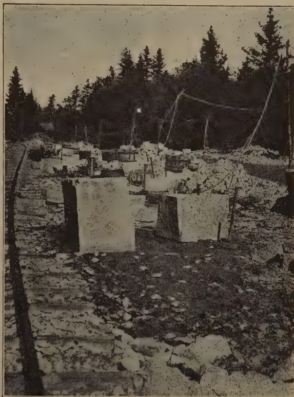
Paving Cutters' Berths with Half Barrels Filled with Chips and Gravel on which the Paving Stone is Finished.—From Vinalhaven, Maine.
