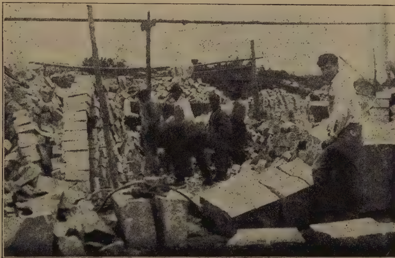
Piles of Finished Paving Blocks. Compressed Air Drilling Machine Resting on Bigger Blocks.—From Lohrville, Wis.
