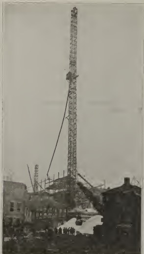
MODERN METHOD OF POURING CONCRETE FOR SKYSCRAPER
