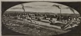
This Is The World's Largest Match Factory; It Is In Sweden
