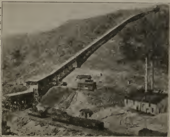
A HILLSIDE COAL MINE
