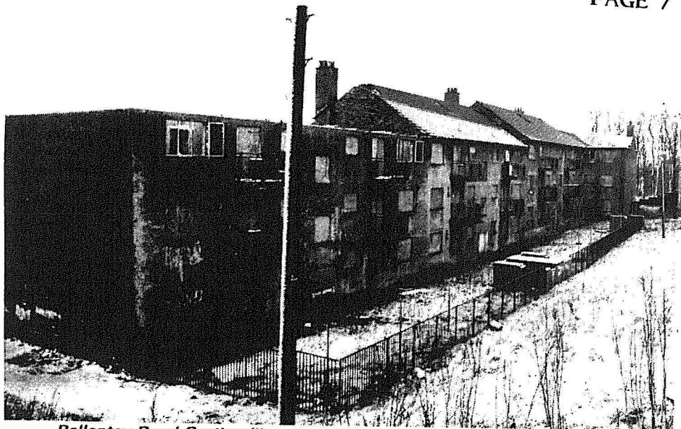
Ballantay Road Castle Milk - one of the areas for co-op renovation.
