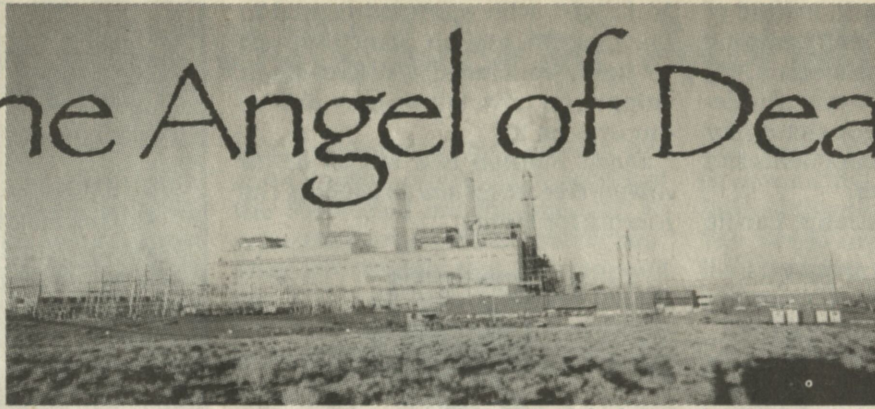
The PNM coal-fired power plant in New Mexico
