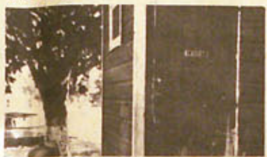
OUT-HOUSE -- NO INDOOR BATHROOMS FOR THE WORKERS.
