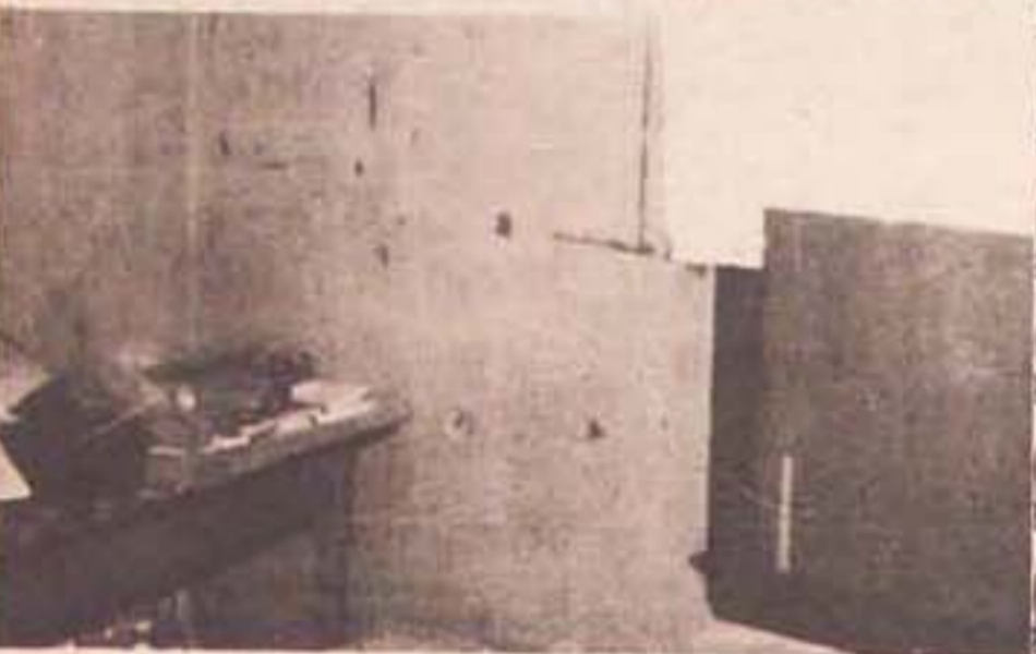
Bullet holes in walls of Ohio, N.C.C.F.
