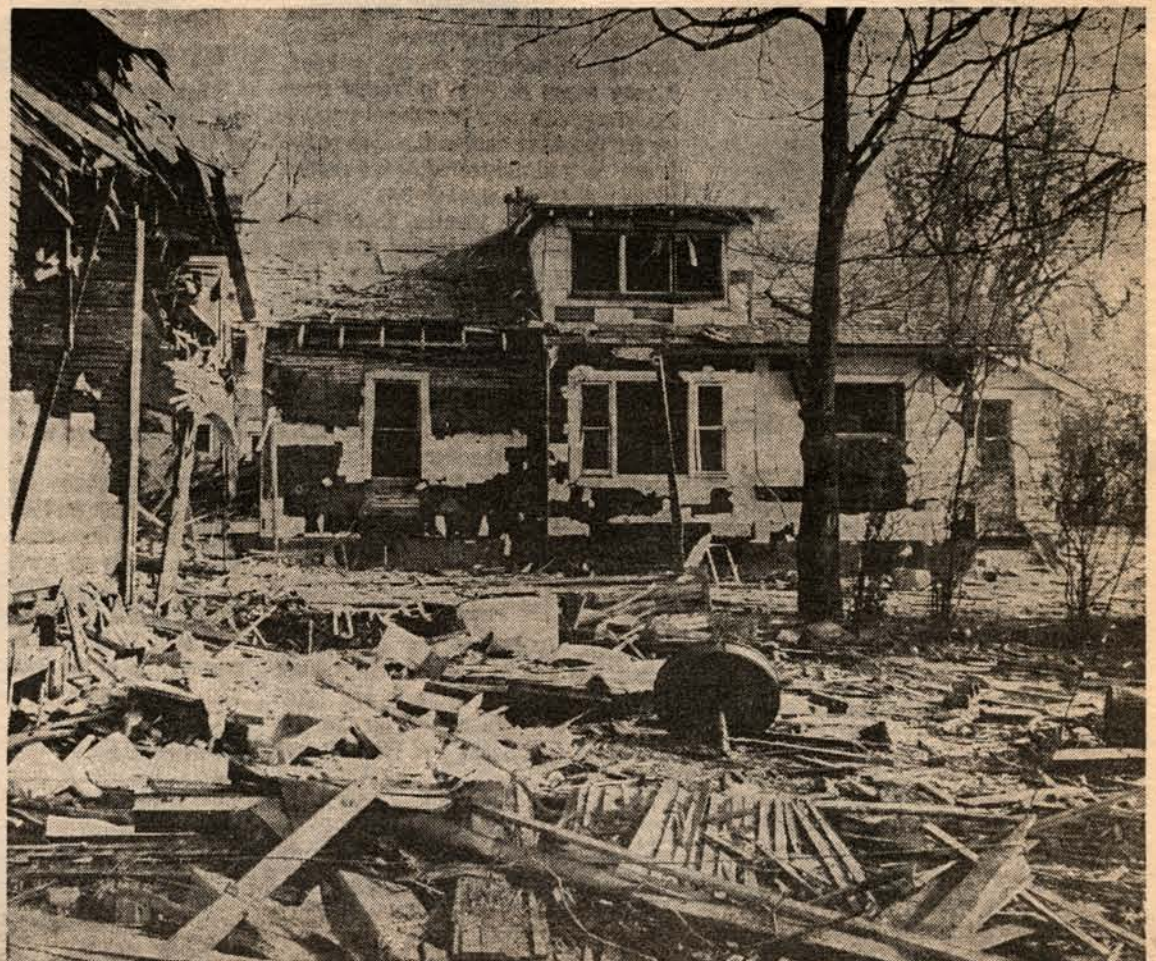
Near by home damaged by blast
