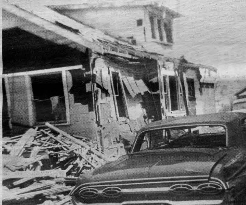
Neighbors auto destroyed with home
