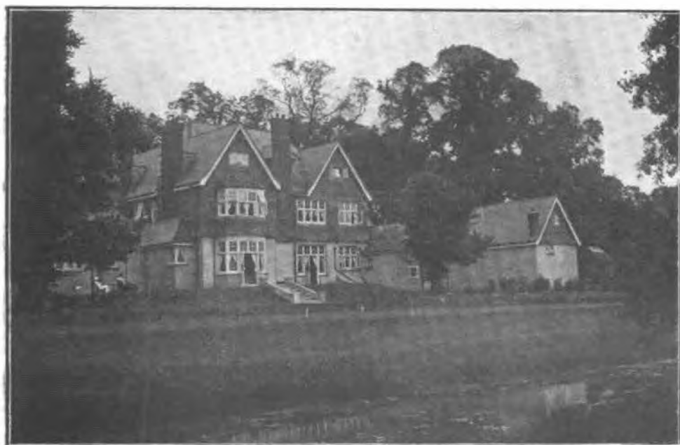
GROVE COURT. VIEW FROM THE GARDEN.
