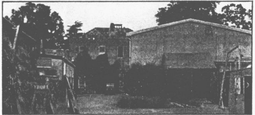
Above: Technical details of Bray Studios from the 1957 Kinematograph Year-book. The photograph shows a section of the Bray country house and Sound Stage No. 2. Bits of set were constructed here to represent the exterior of the prison in THE CURSE OF FRANKENSTEIN.
