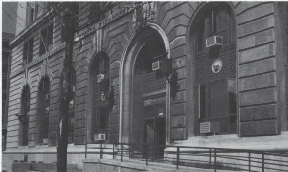
Detroit Police Headquarters, 1300 Beaubien. It was inside these walls that Dutch took his advanced studies in homicide and police procedure.
