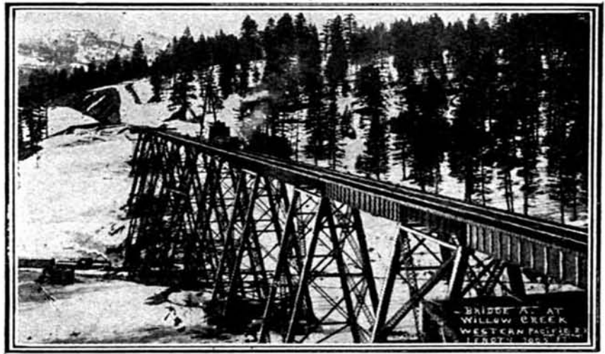
A Trestle Bridge
